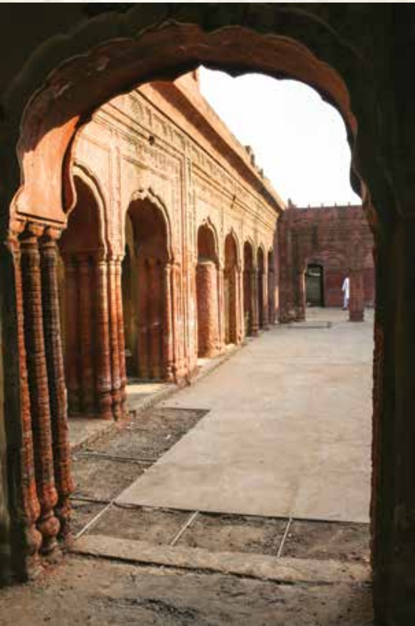
One of the cusped arches.
